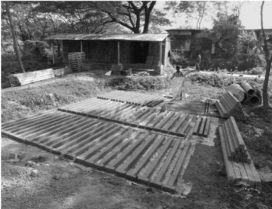
FIGURE 6. Prefabricated RCC columns are sold in the local market.
