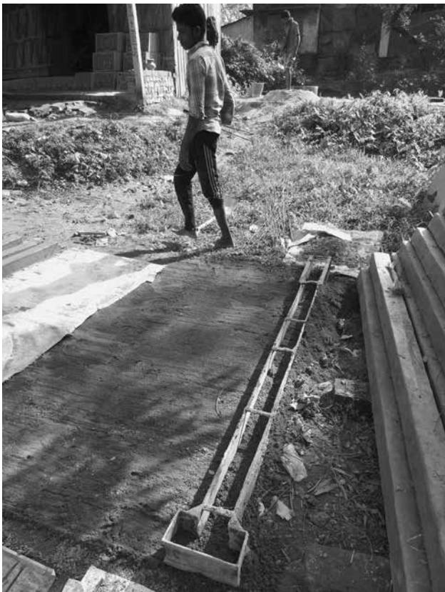
FIGURE 7. Mold used in the making of prefabricated columns.
