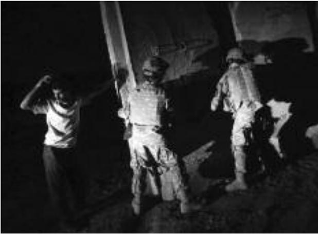
**FIGURE 8.** MNF soldiers worked through the night using a crane to lower concrete 14,000-pound blast wall segments between Shi'a and Sunni neighborhoods in Dora. Photo by Chris Hondros/Getty, posted online at [http://iraqlogger.powweb.com/fullimage.php?img=75030515\\_10.jpg](http://iraqlogger.powweb.com/fullimage.php?img=75030515_10.jpg), accessed February 1, 2010.
