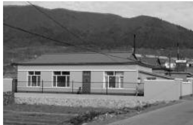
FIGURE 16. Newly built houses for ethnic Koreans in Yueqing Township in 2007 as part of the state-led project of constructing socialist new rural communities. The glazed windows and color scheme altogether change the traditional appearance of the Korean-Chinese house.
