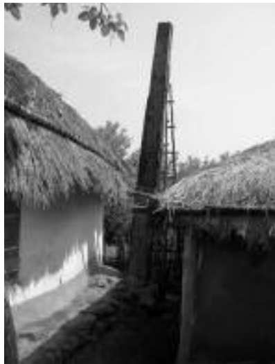
FIGURE 10. A Korean-Chinese chimney (Lutian Village) is built as a diminutive tower with a square vertical pipe, and is placed beyond the end-wall of the house.
