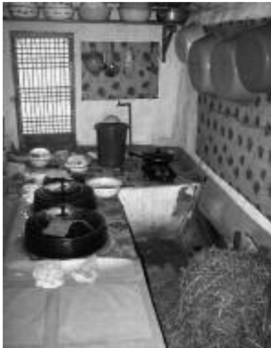
FIGURE 3. Three fire holes and the fire pit in the kitchen of a Korean-Chinese house in Lutian Village.
