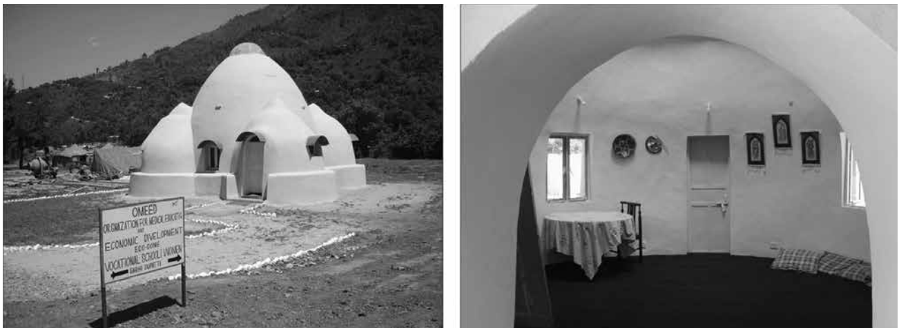
FIGURE 11. Vocational Institute at Garhi Dupatta near Balakot, built using Cal-Earth technology. Images downloaded from FaceBook with OMEED's permission.
