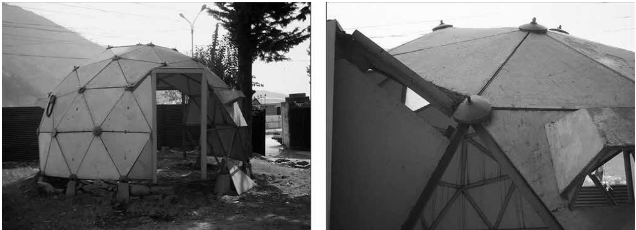
FIGURE 10. Experimental geodesic dome in Balakot. Photo by Mohammad Ashraf Khan.
