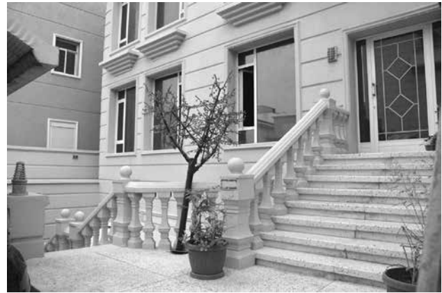
FIGURE 14. F.D.'s separate entrances to house and basement. Photo by author, 2016.
