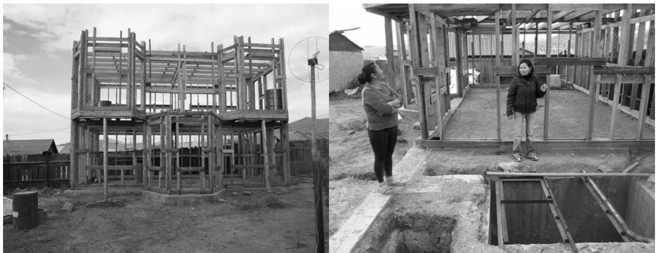
FIGURE 4. Foundations and framing for this home were inspired by a Canadian house seen on television. A son learned to use computer-aided drafting software with sufficient proficiency to lay out a design with more forethought than most ger -district houses. Forethought was also key to staging construction as family savings accrued over time. At the time of the photo, the family had purchased cladding material and were planning to restart construction to complete the exterior. They calculated that completion would likely require a subsequent summer.
