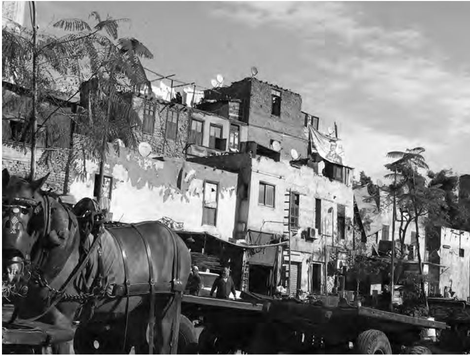
FIGURE 13. Houses left undemolished in the Ishash al-Tourguman area. Photo by author.
