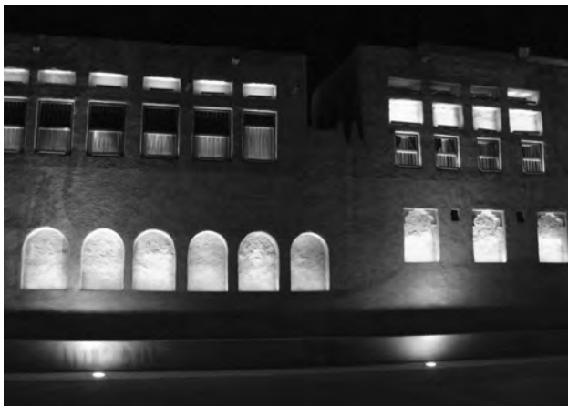
FIGURE 9. Boutique lighting at the Majlis Gallery.
