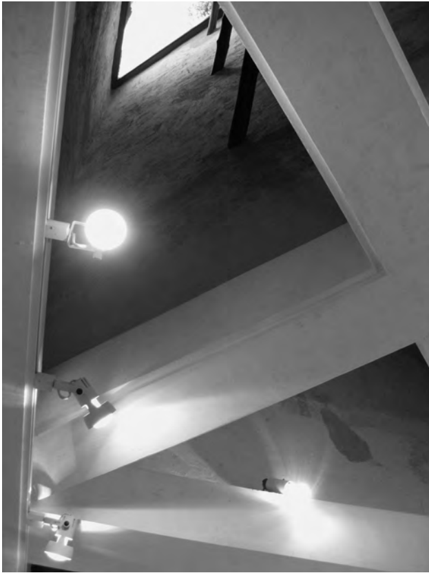
FIGURE 12. Wind tower used for gallery lighting at the Majlis Gallery.
